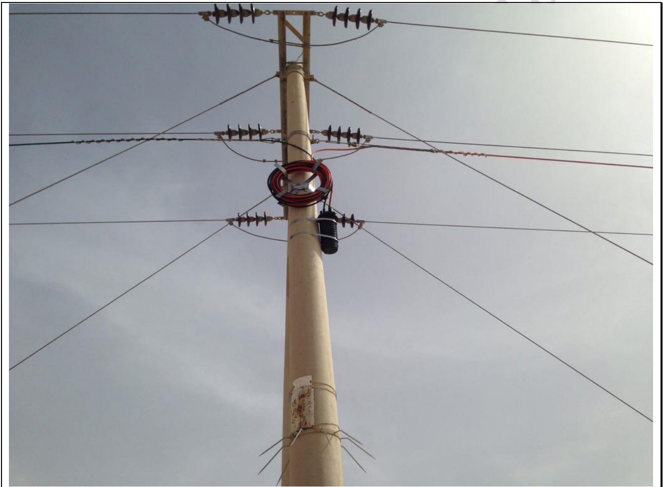
Aerial Cable Storage Configuration With Cross-bar
